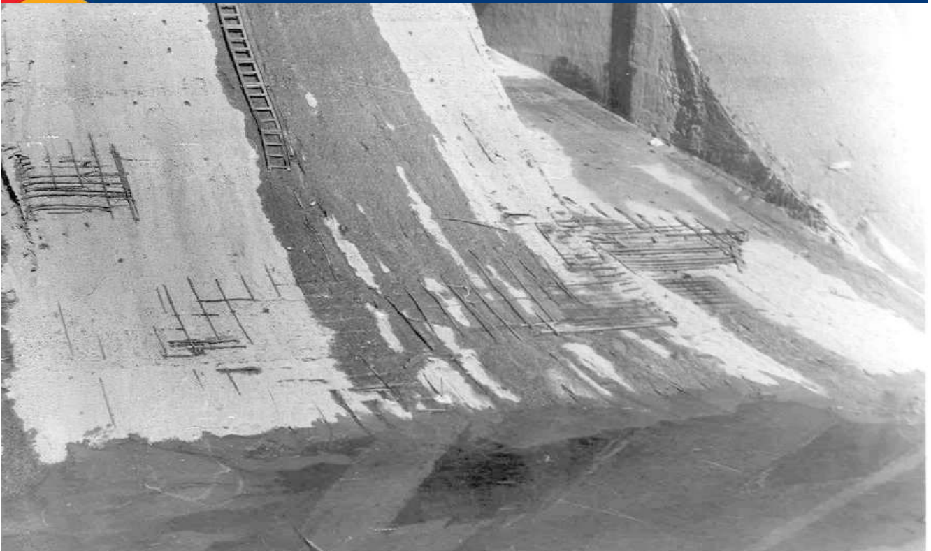
EROSION IN SPILLWAY GLACIS-1996 SALAL HE PROJECT
