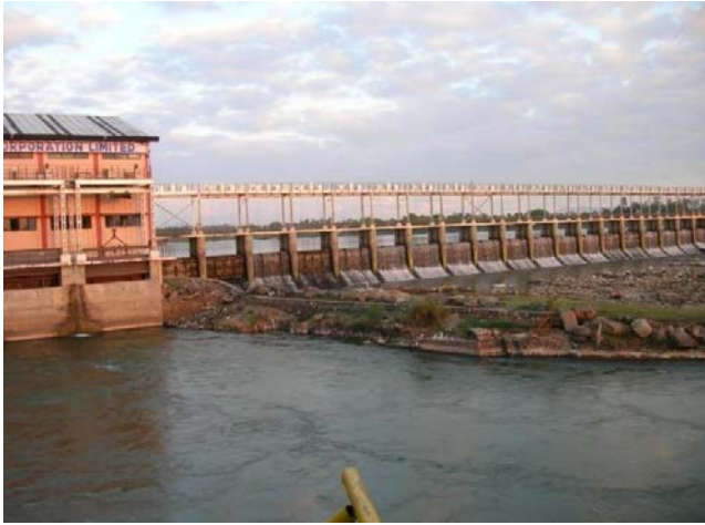
Low head power plant (4.5MW) Madhavmantri, (head 4.5 m) Kaveri River, India
