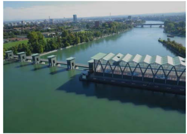
Low head power plant (90 MW) BIRSFELDEN, (head 3 to 9 m) Rhine river, Switzerland
