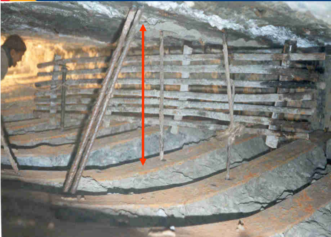
DAMAGED UNDERSLUICES
