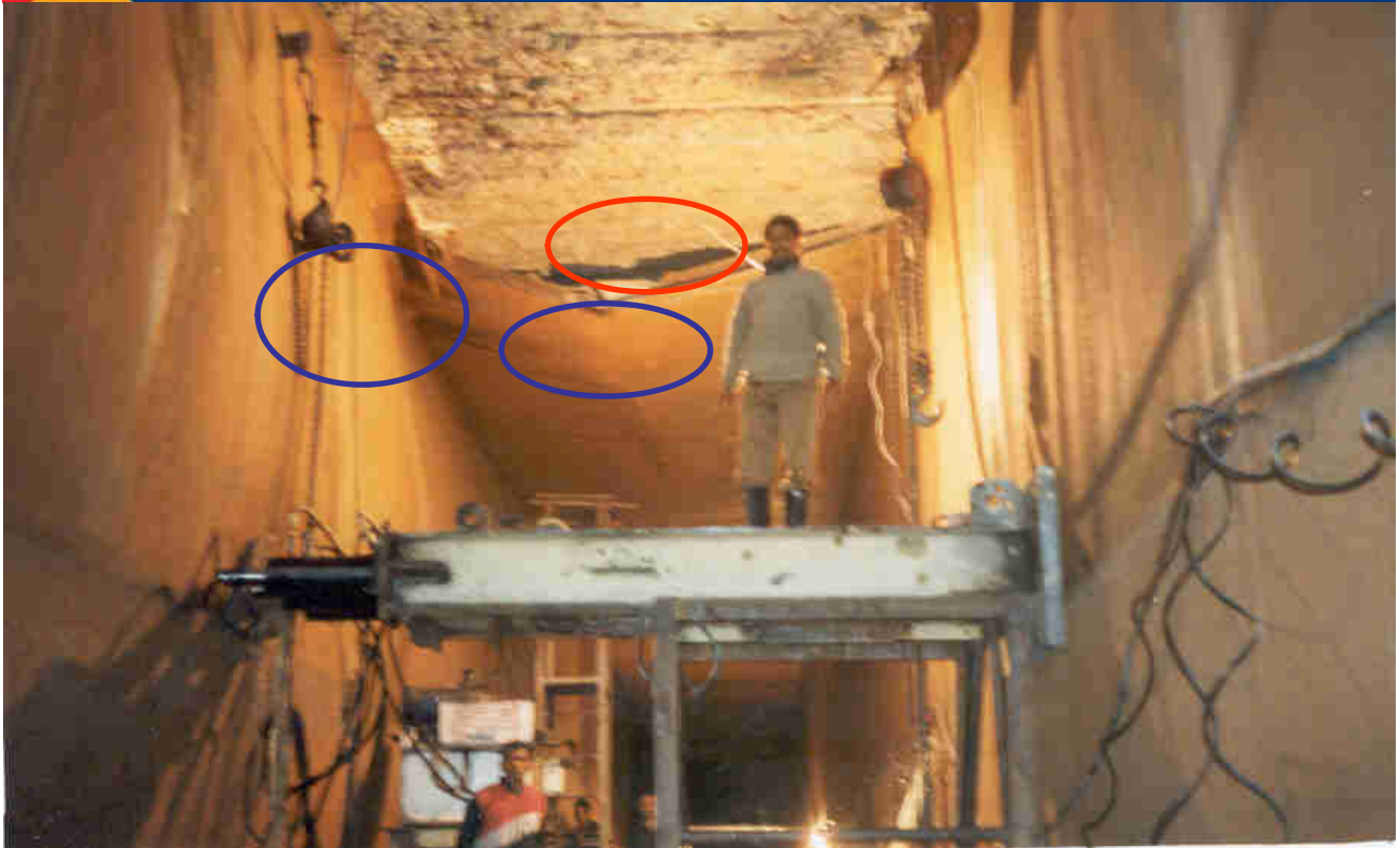
DAMAGED UNDERSLUICES IN CHAMERA DAM
