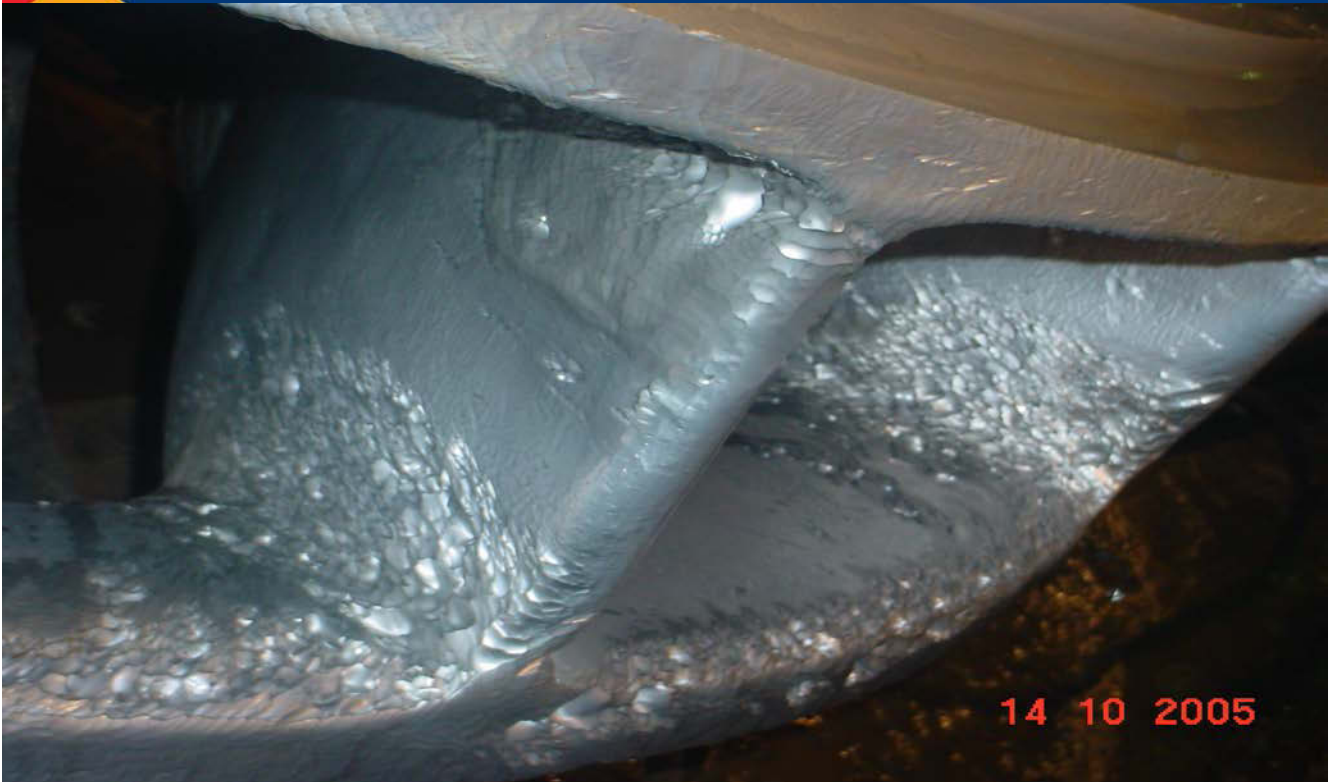
Damaged Runner photographs of Unit #1 taken out during 2005-06 maintenance BAIRA SIUL H.E. PROJECT
