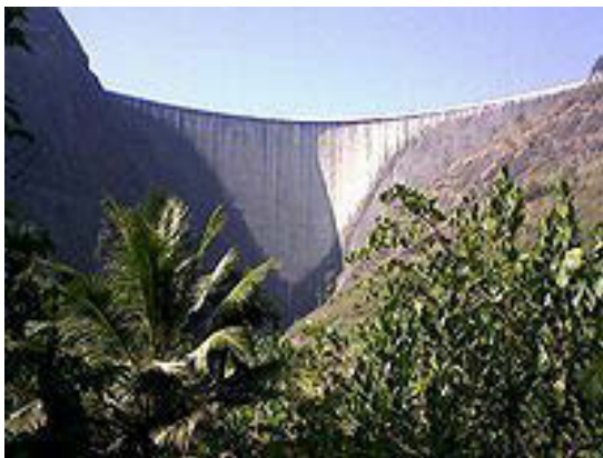
Double Curvature Arch Dam, Idukki.
