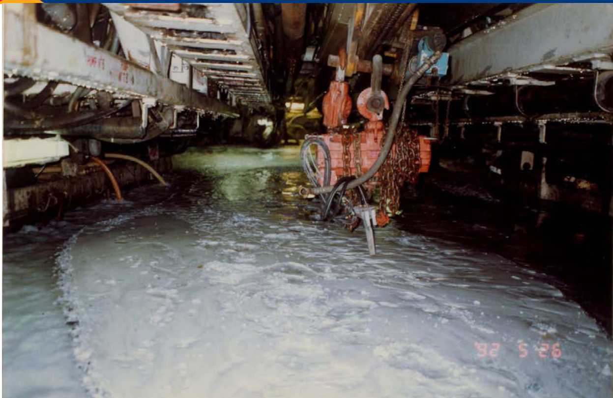
Muck Deposit due to High Ingress of Water in HRT
